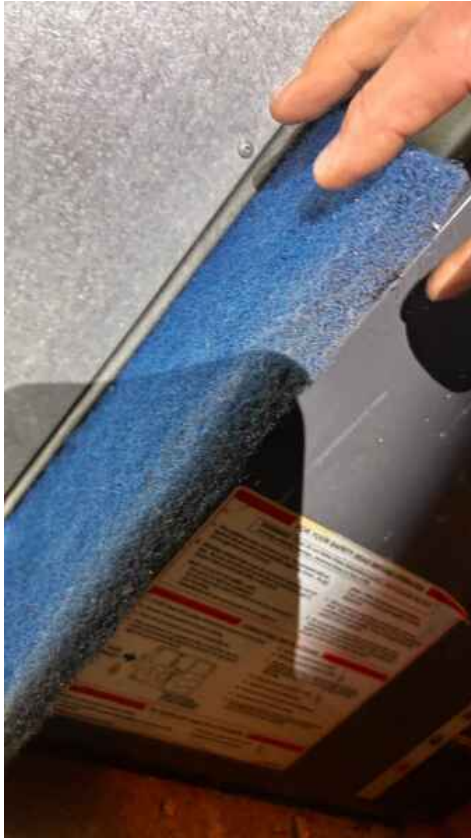
Upgrade filter and change regularly
