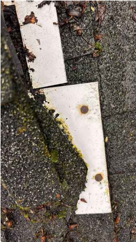
Exposed Fasteners
