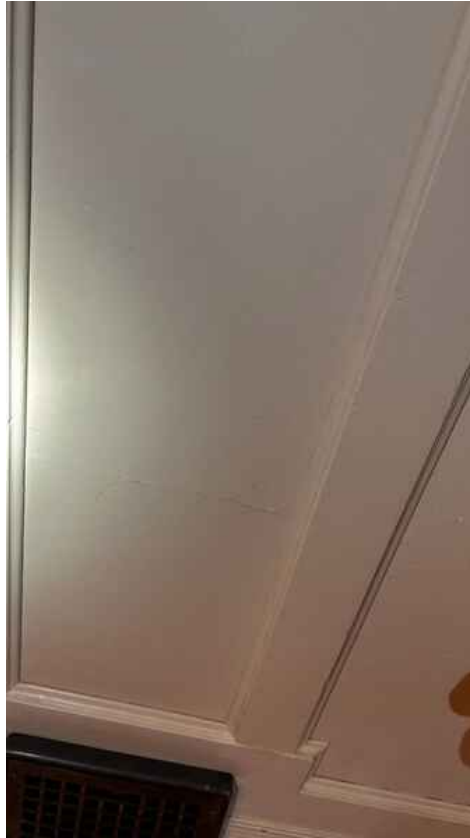
Cracked paneling
