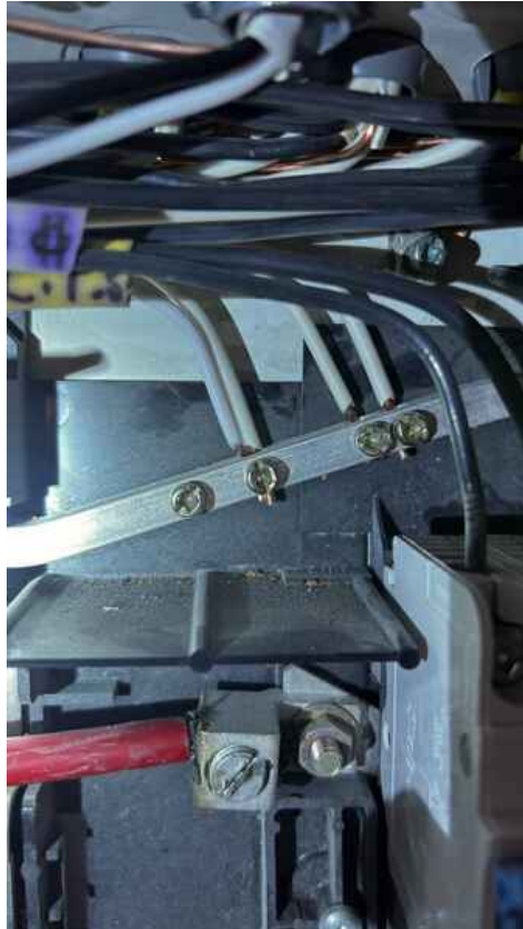
Double tapped neutral (may be ok, depends on panel specs)
