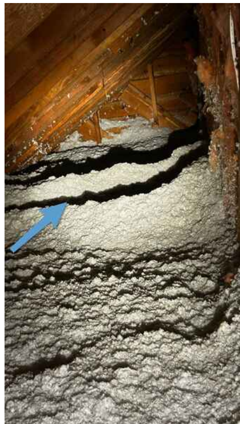
Displaced Insulation
