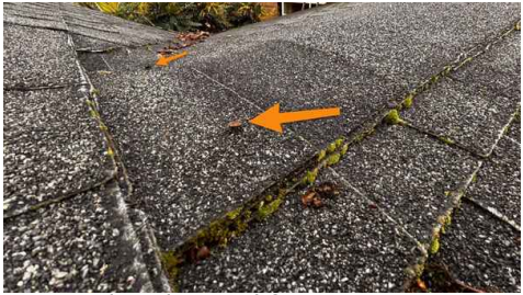
Exposed and proud fasteners
