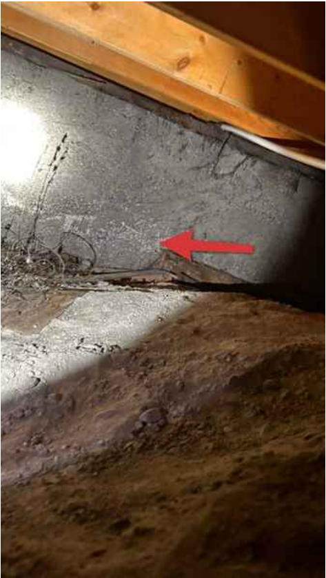
Minor efflorescence
