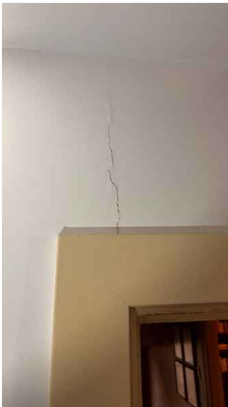
Bathroom door wont close
