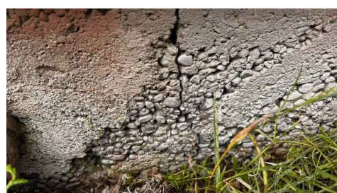
Crack + Honeycombing
