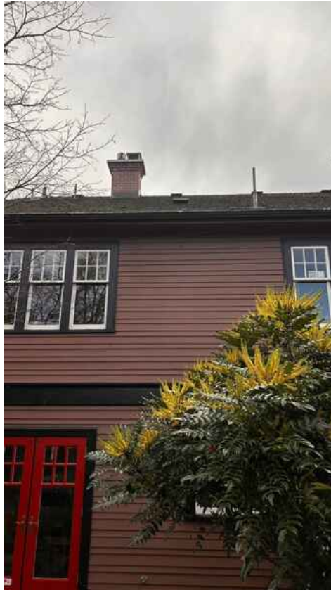
Trim Tree back to 3ft of clearance
