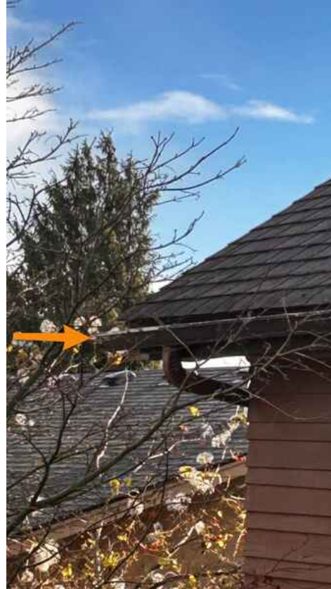
Loose/Leaning Gutter
