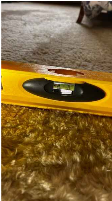
Level Showing floor displacement
