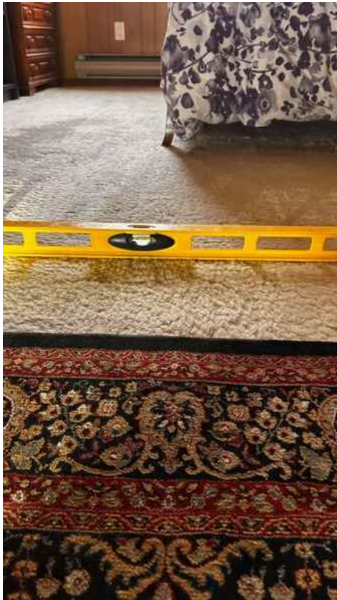
Floor displacement
