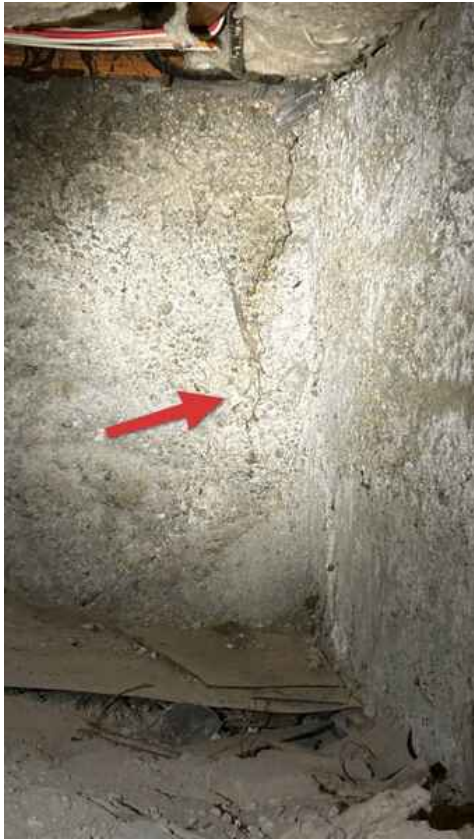
Foundation crack
