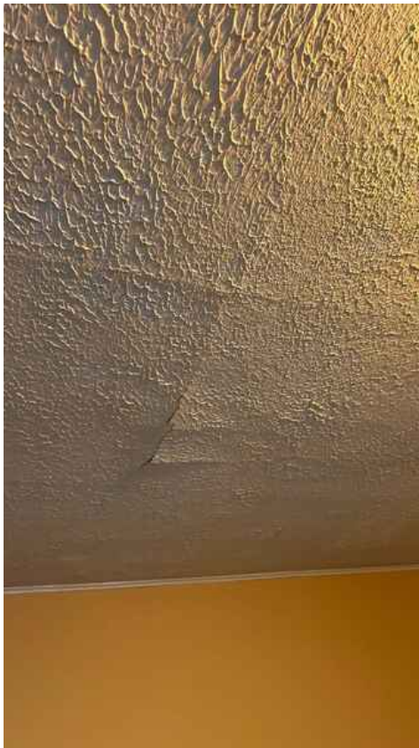
Cracked plaster
