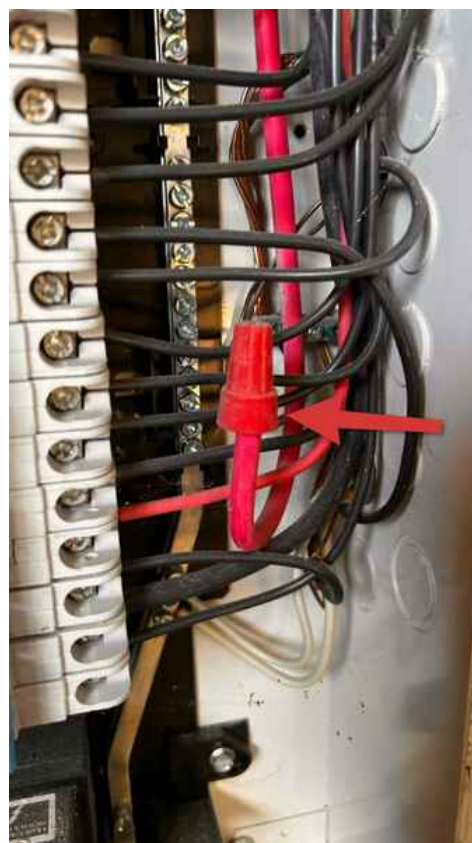
Terminated Conductor
