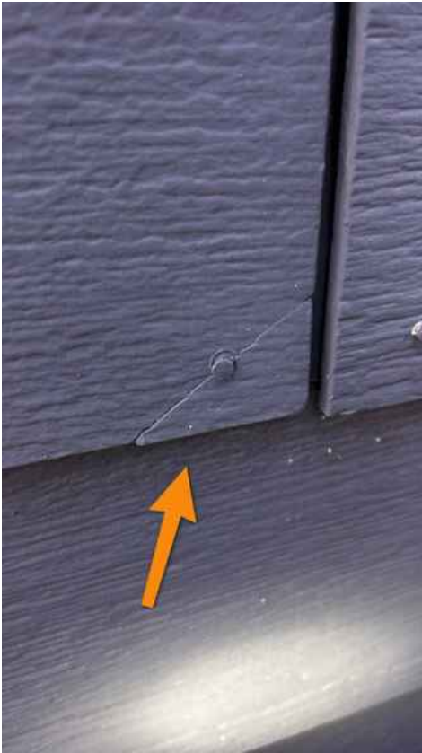
Cracked siding
