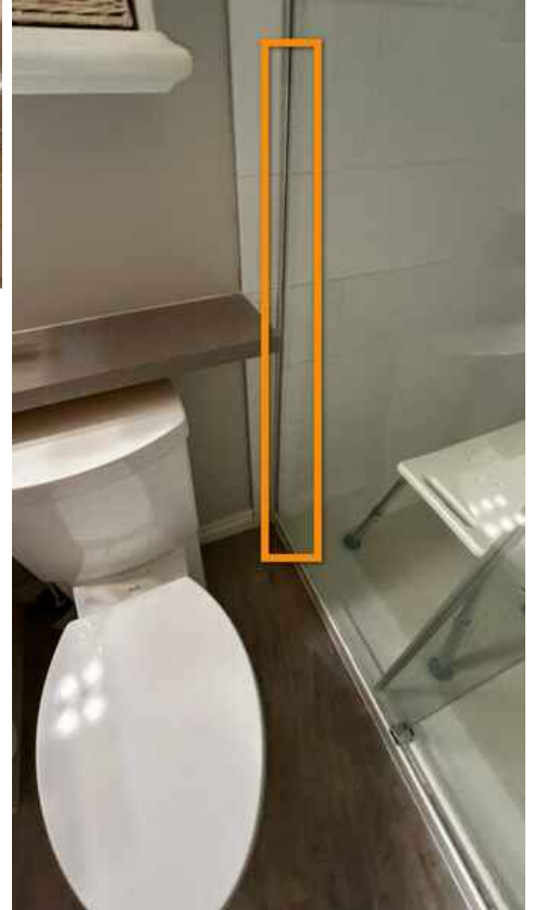
Seal Wall to Tile to prevent leaks
