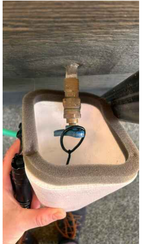
Upgrade Hose Bibs
