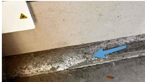
Efflorescence
