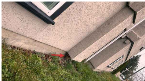
Cast Iron Drain & Waste
