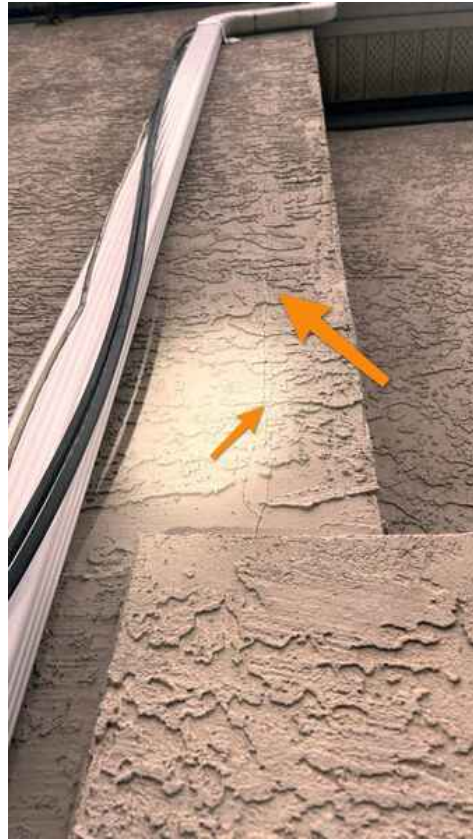
Stucco cracks
