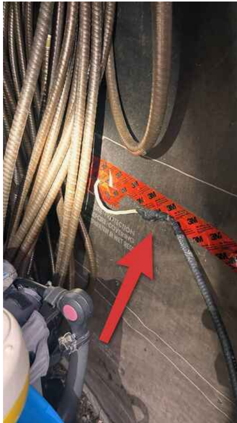
Improper connection
