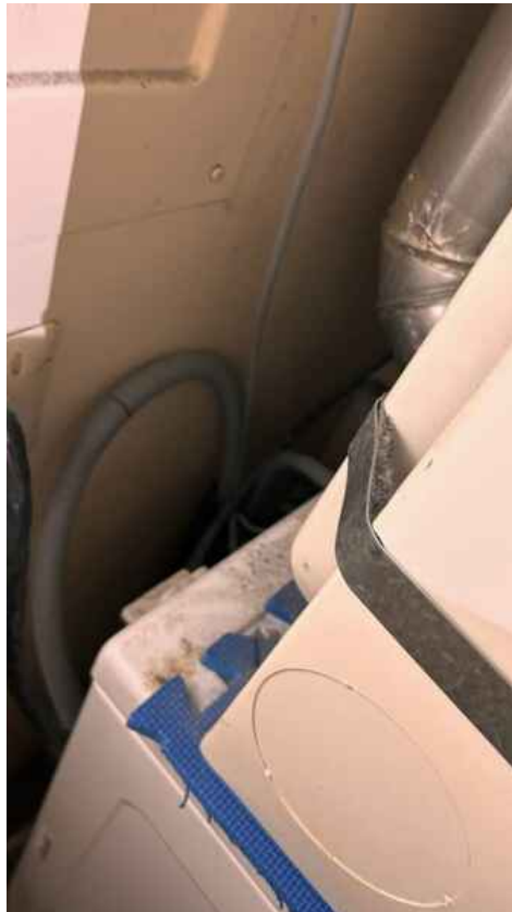
Upgrade Laundry hoses to steel braided
