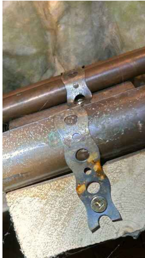
Different metals shouldn't be touching
