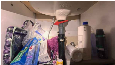
Possible Poly-B (easy upgrade to steel braided hoses)
