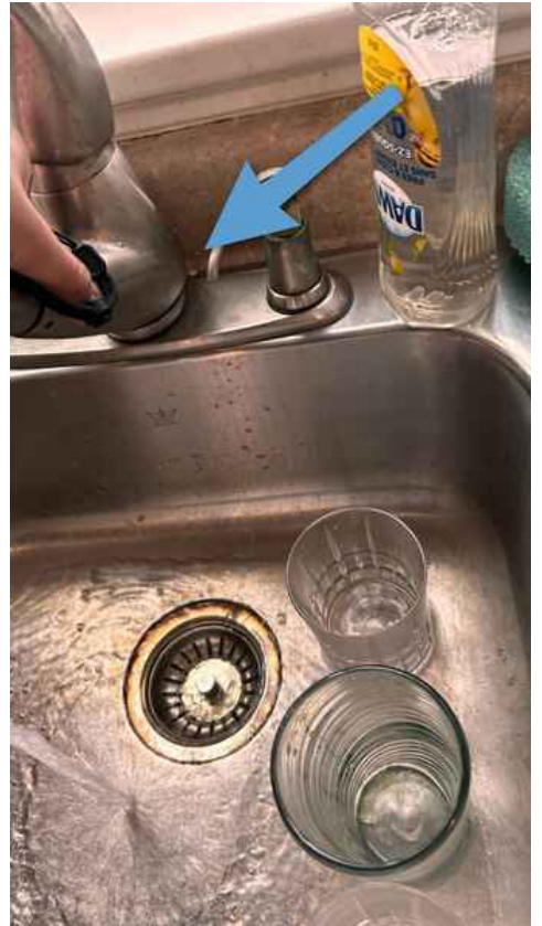
Loose faucet assembly
