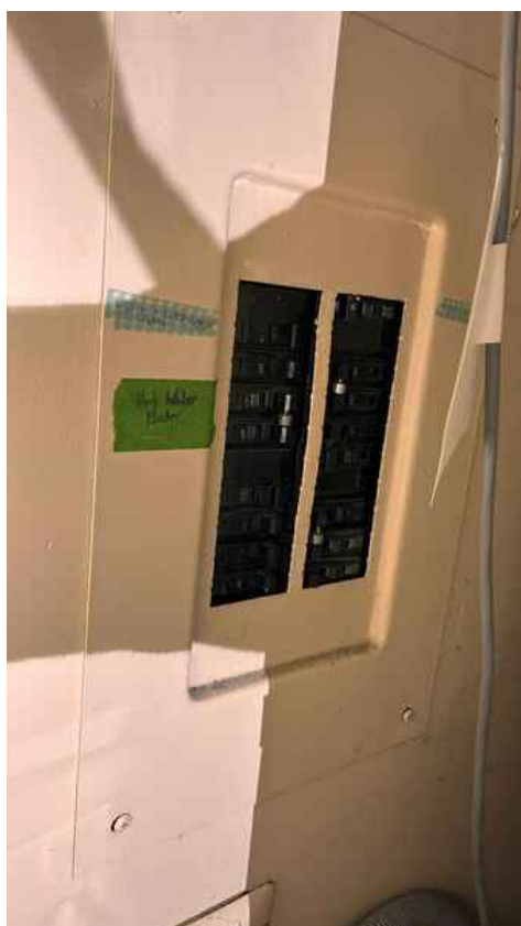
Inaccessible Panel (behind washer and dryer) Unit A
