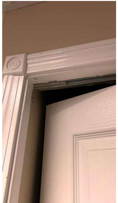
Utility closet off track
