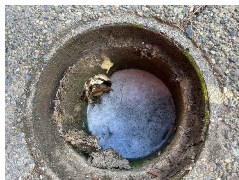
Add 90 degree elbow to improve drain function
