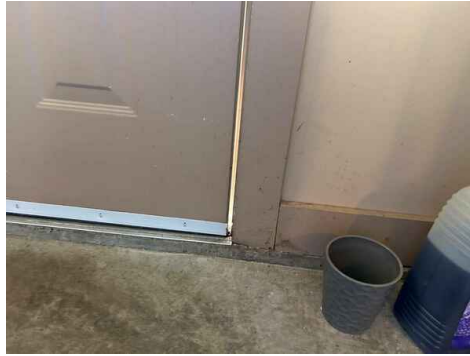
Visible Light through weather stripping
