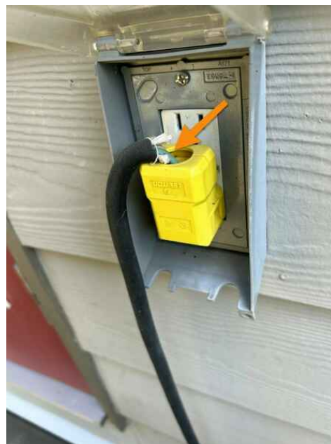
Damaged Cable
