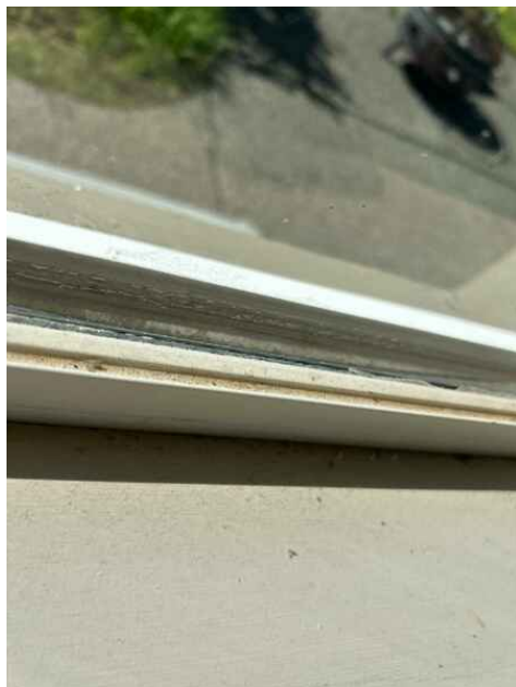
Spacer Deterioration
