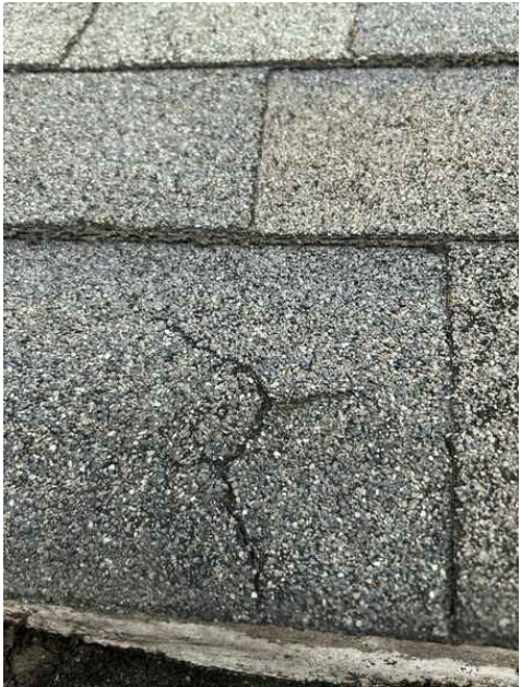
Cracked Shingle
