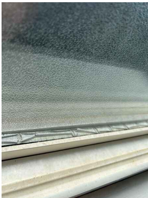
Peeling Spacer Material
