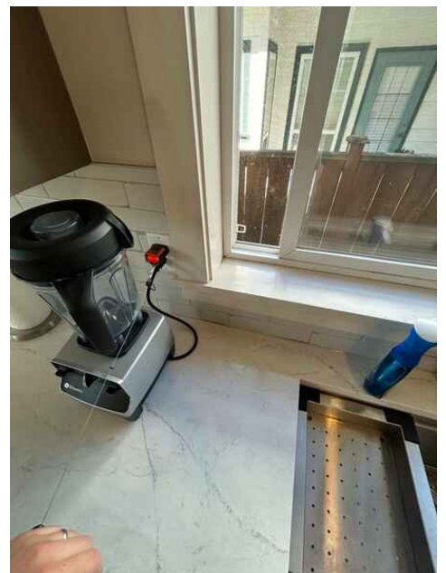
Receptacle Not GFCI
