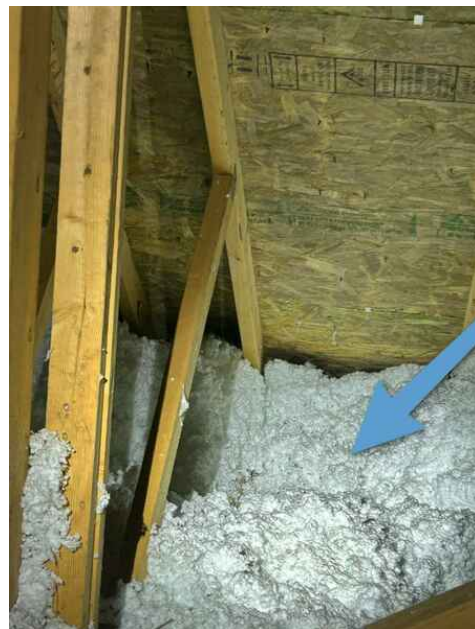
Displaced/Uneven Insulation
