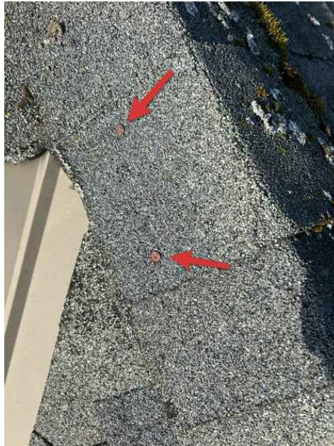
Exposed Fasteners
