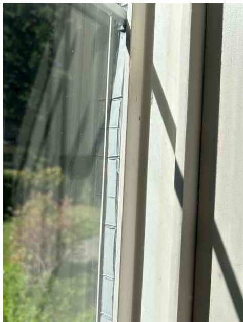
Spacer Damage
