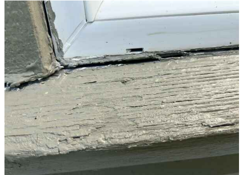
Caulk window gaps
