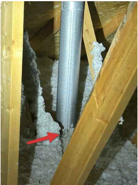
B-Vent requires 1 inch of clearance
