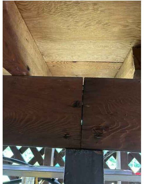
Insufficient Overhang
