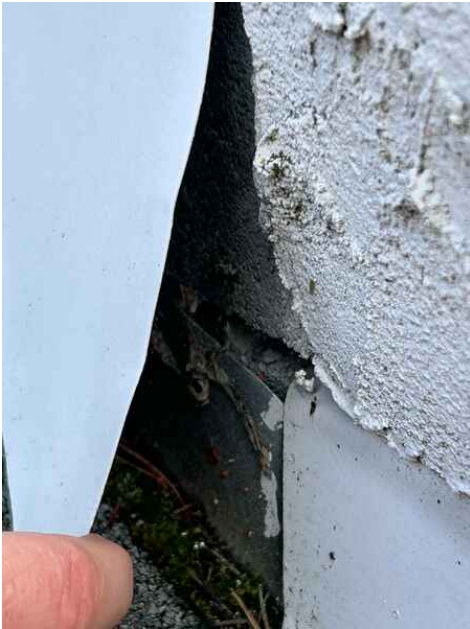
Wind driven rain could enter
