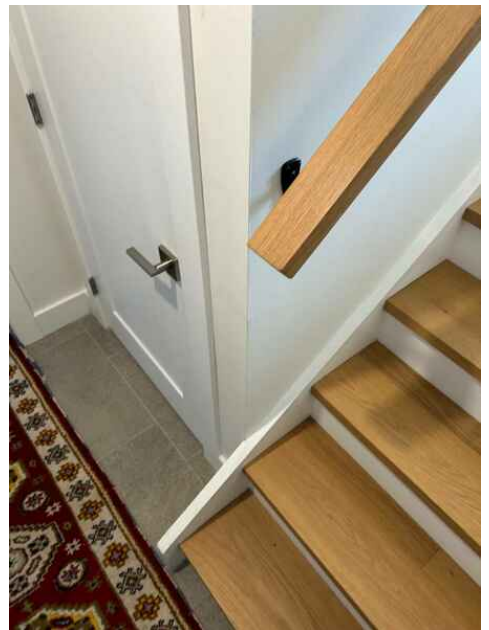
Hand rail doesn't extend
