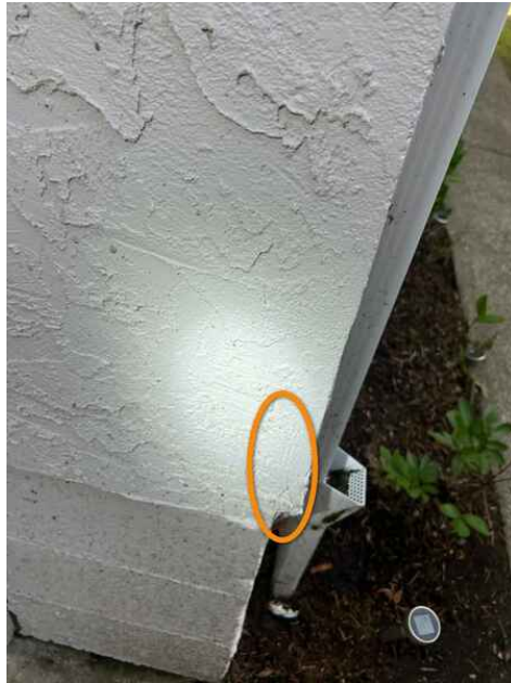
Patch Cracks
