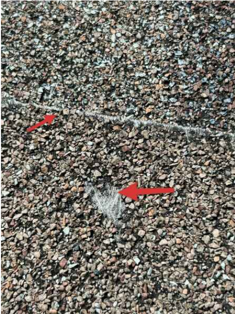
Fiberglass matt showing
