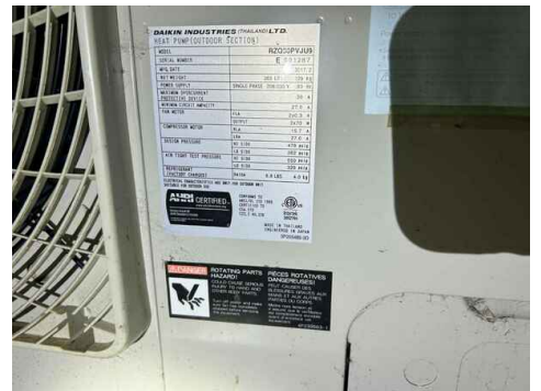
Heat pump data plate
