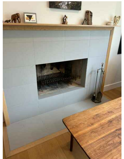
WETT inspection required
