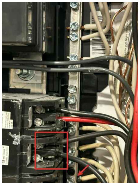
Aluminum Wiring
