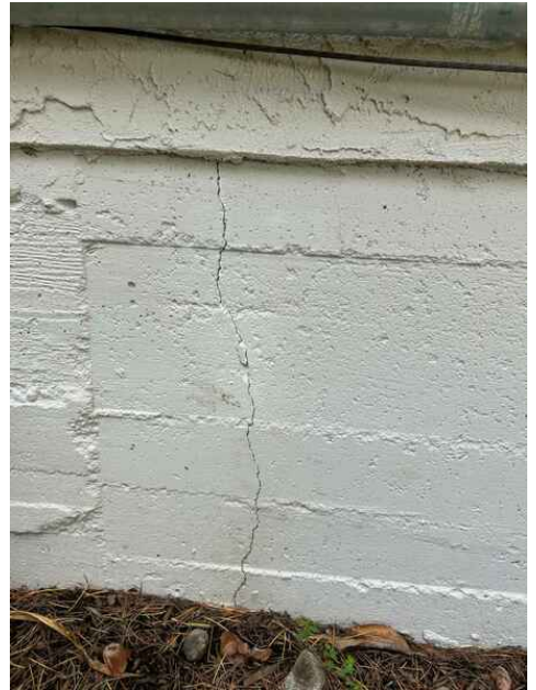
Foundation Crack
