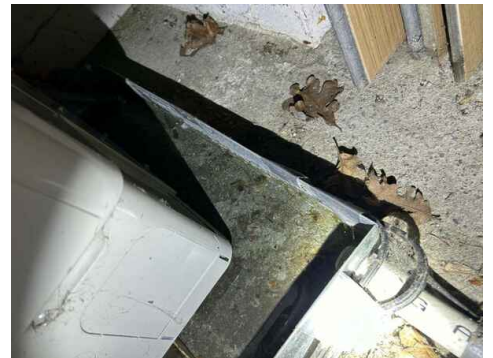
Permanently flooded pan
