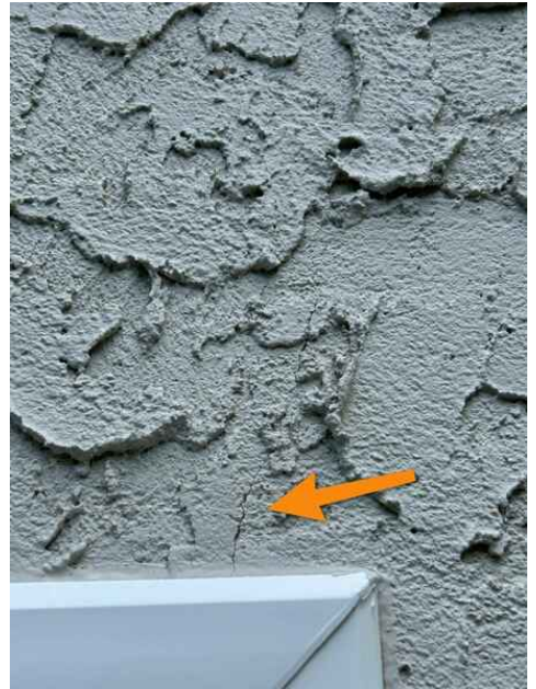
Patch Cracks
