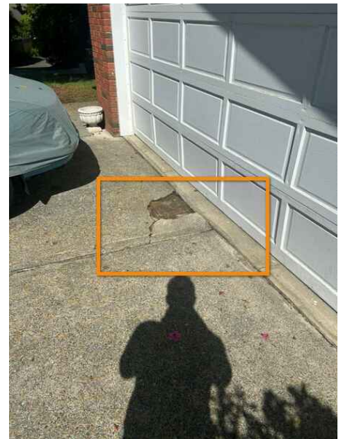
Upgrade old drain to a slot style drain\
