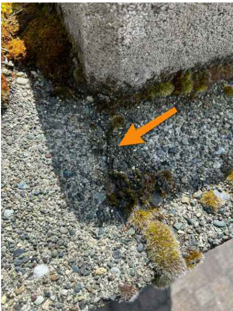
Cracked Crown
