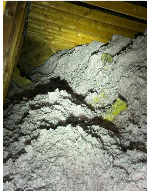
Compressed insulation
