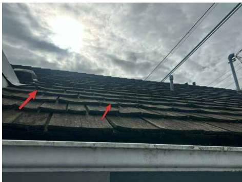
Multiple sections are cupping and lifting
