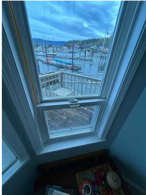
Hung window needs to be pushed a certain way to close
