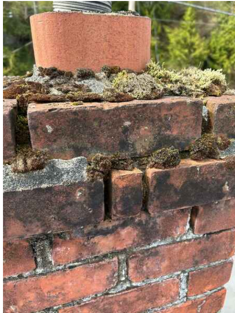
Repoint of mortar and possible rebuild needed
