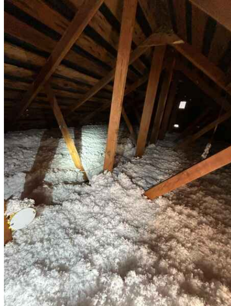
Irregularly spaced rafters
