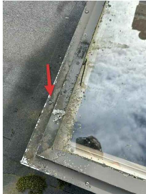
Exposed hardware on skylight, evidence of water pooling
