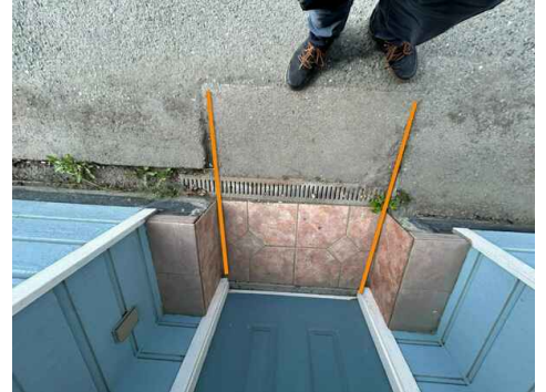
Grade towards home and low threshold on entry door
