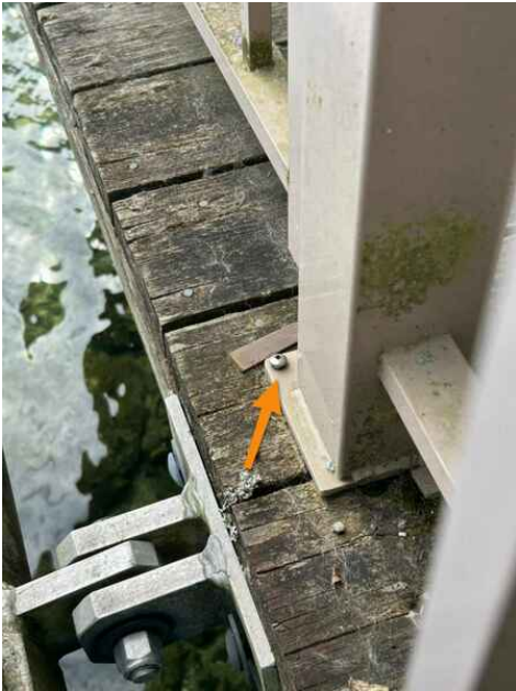
Hardware drilled into surface
