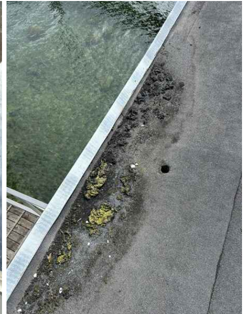
Pooling evidence = Drainage issues
