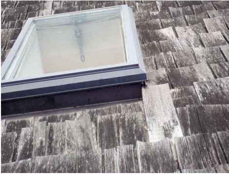
Skylight built on curb
