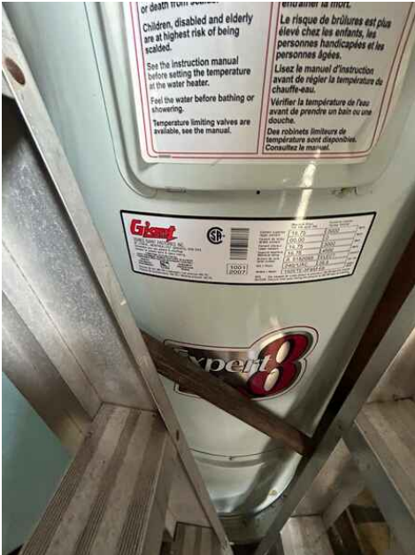
No seismic straps
