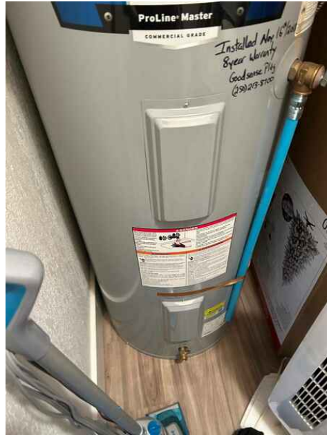
No seismic straps/drip pan
