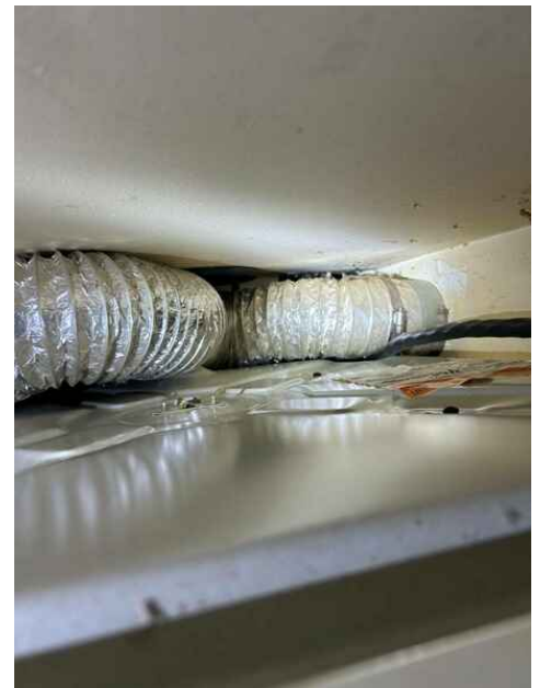
windy dryer vent material
