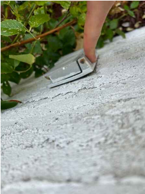
Exterior aged outlet not GFCI protected Kitchen receptacle near sink not GFCI
