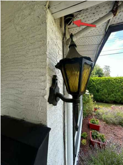
Steel Wool used as deterrence
