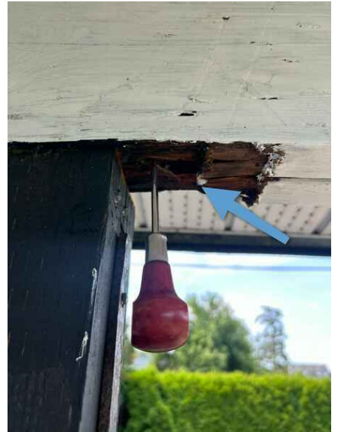
Paint exposed beam
