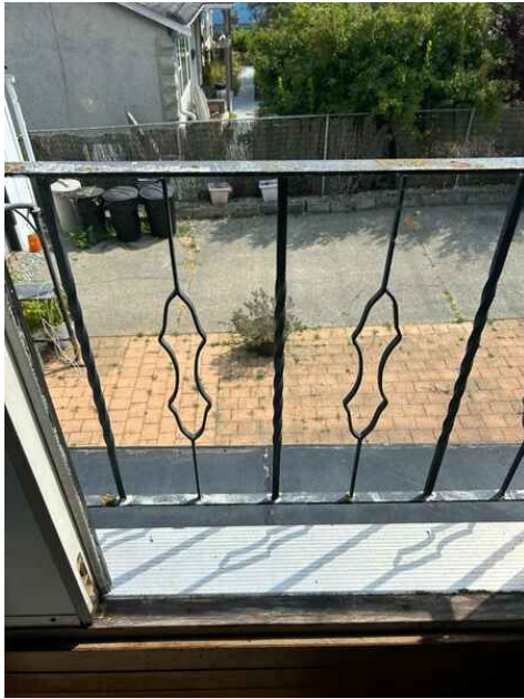
Wide Balusters, Short Guard Rail
