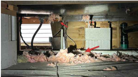
Exposed Belly/ Torn insulation
