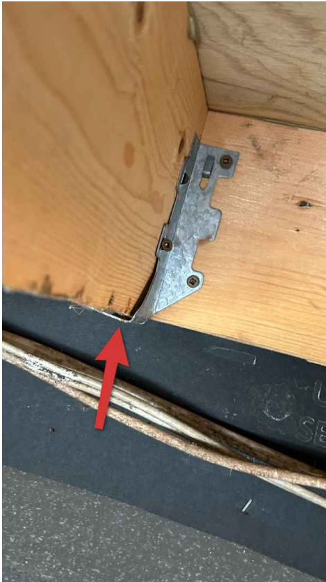
Floating Joist
