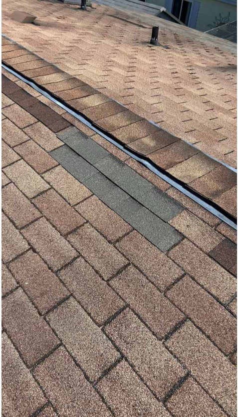
Different Product Indicating Possible Previous Leaks
