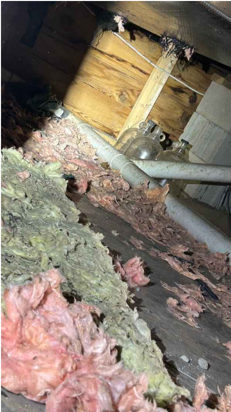
Insulation Shredded
