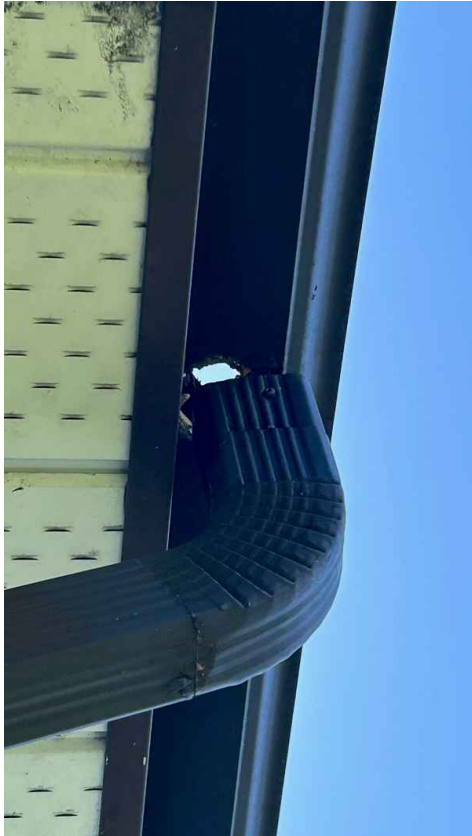
Misaligned Downspout
