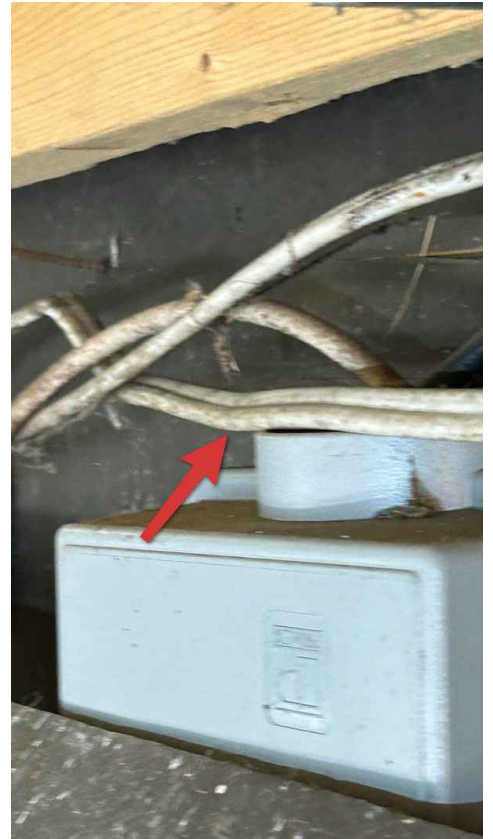
Conductors used outside must be rated for exterior
