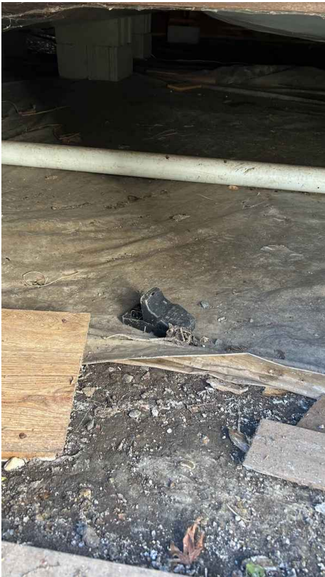
Incomplete vapor barrier
