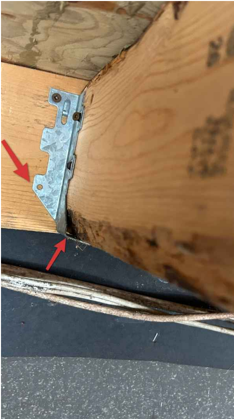
Missing Fasteners
