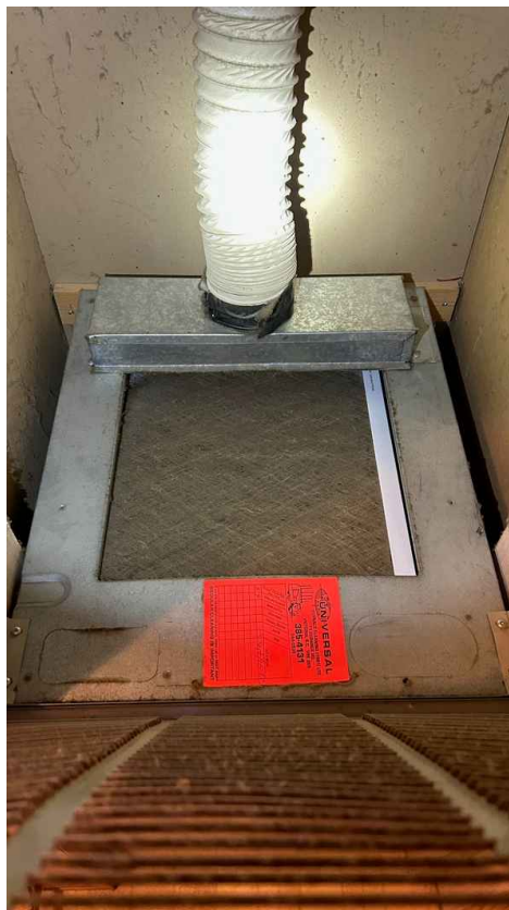
Improper venting material, Very dusty components and filter
