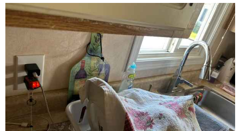
Kitchen outlet not GFCI protected
