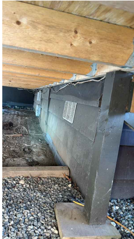
Deck using home for support
