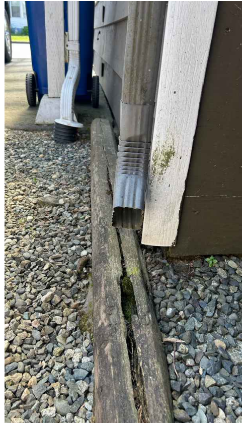
Downspout Draining too close to home
