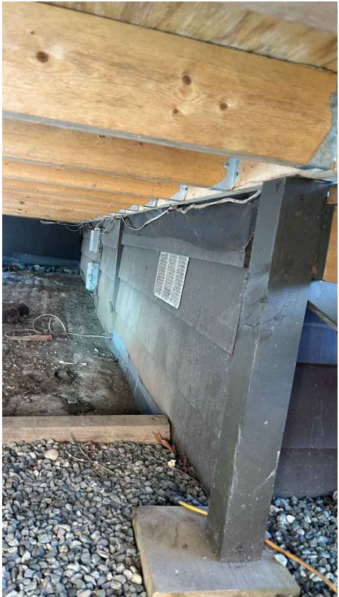
Deck Attached to Manufactured Home
